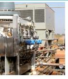
Used as: ↗ Multiphase pump Gas volume fraction: **∧** GVF = 56 % Flow rate: ↗ Q = 395-1,000 m³/h [1,739-4,402 GPM] Differential pressure: ↗ △P = 7.3- 56.2 bar [105-915 psi]
