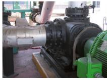
Used in: **↗** Fuel oil power plants Pumped liquid: ↗ Heavy fuel oil Flow rate: ↗ Q = 876 m³/h [3,857 GPM] **Differential pressure: ∧** AP = 48 bar [696 psil]
