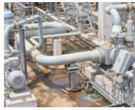
Used in: ↗ Tank storage in Singapore Pumped liquid: ↗ Various black and white products Flow rate: ↗ Q = 2,000 m³/h [8,806 GPM] Differential pressure: **∧** ΔP = 11 bar [160 psi]
