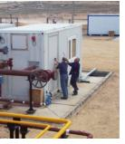
↗ Multiphase pump Gas volume fraction: **7** GVF = 86.6 % Flow rate: ↗ Q = 175 m³/h [770 GPM] Differential pressure: **∧** ΔP = 38 bar [551 psi]
