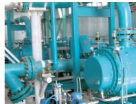
Used as: ↗ Pipeline booster pumps Pumped liquid: ↗ Crude oil Flow rate: ↗ Q = 180 m³/h [793 GPM] Differential pressure: **∧** ΔP = 60 bar [870 psi]
